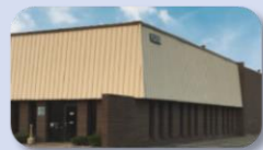
Dearborn, MI Manufacturing and engineering facility
